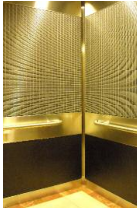
William Penn House: lower panels in Black Quartz; upper panels in GageCast Woven Linear; Satin SS accent panels; 1.5" tubular handrail
