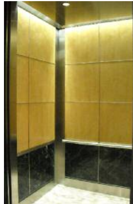
1515 Wynkoop: lower panels in Verde Antique stone; upper panels in Curly Maple wood veneer; inlay in Satin SS; Custom Satin SS ceiling with LED perimeter lighting; custom handrail
